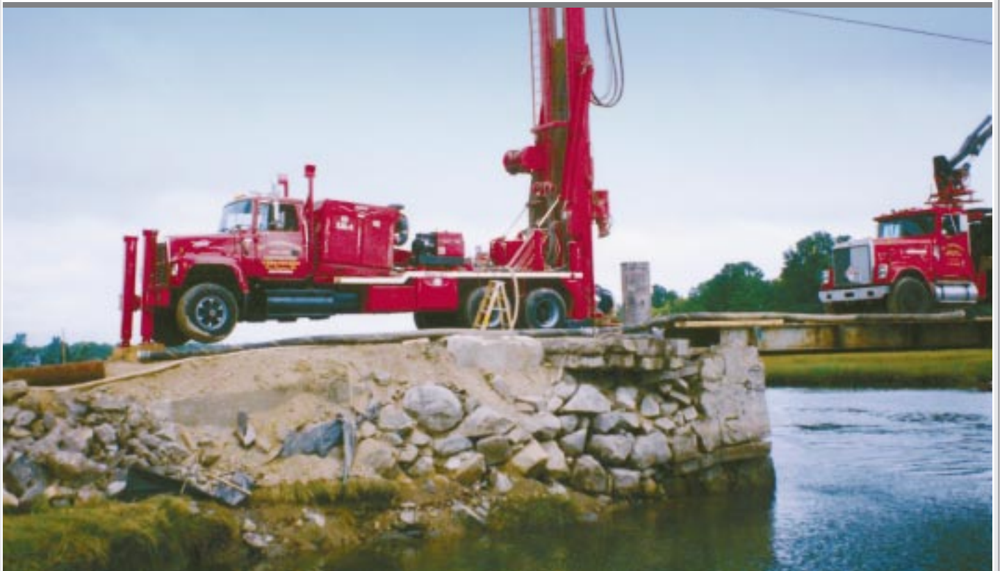
Retrofitting bridge foundation piles with Foremost DR-24
