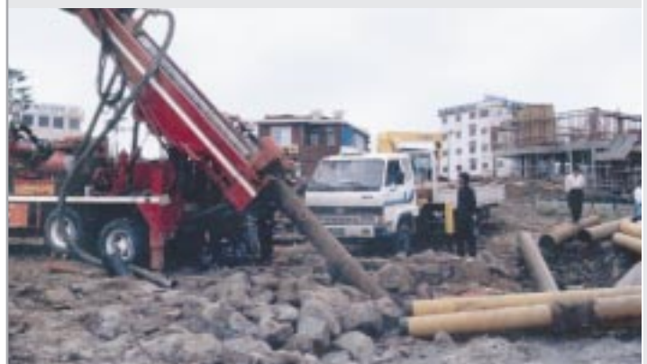
Foremost DR-24 drilling and casing at 45-degree angle
