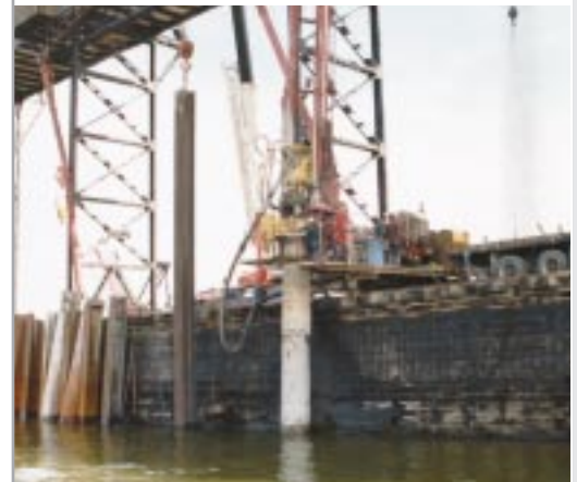
Below - DR-40 drilling rock-socketed holes for grouted H-beams on wharf construction
